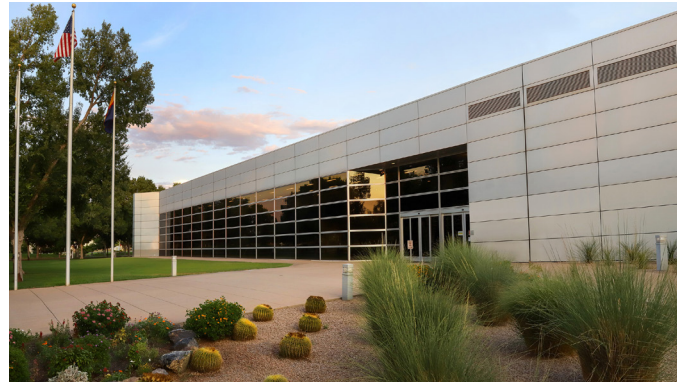
NXP's high-volume GaN manufacturing facility in Chandler, Arizona
