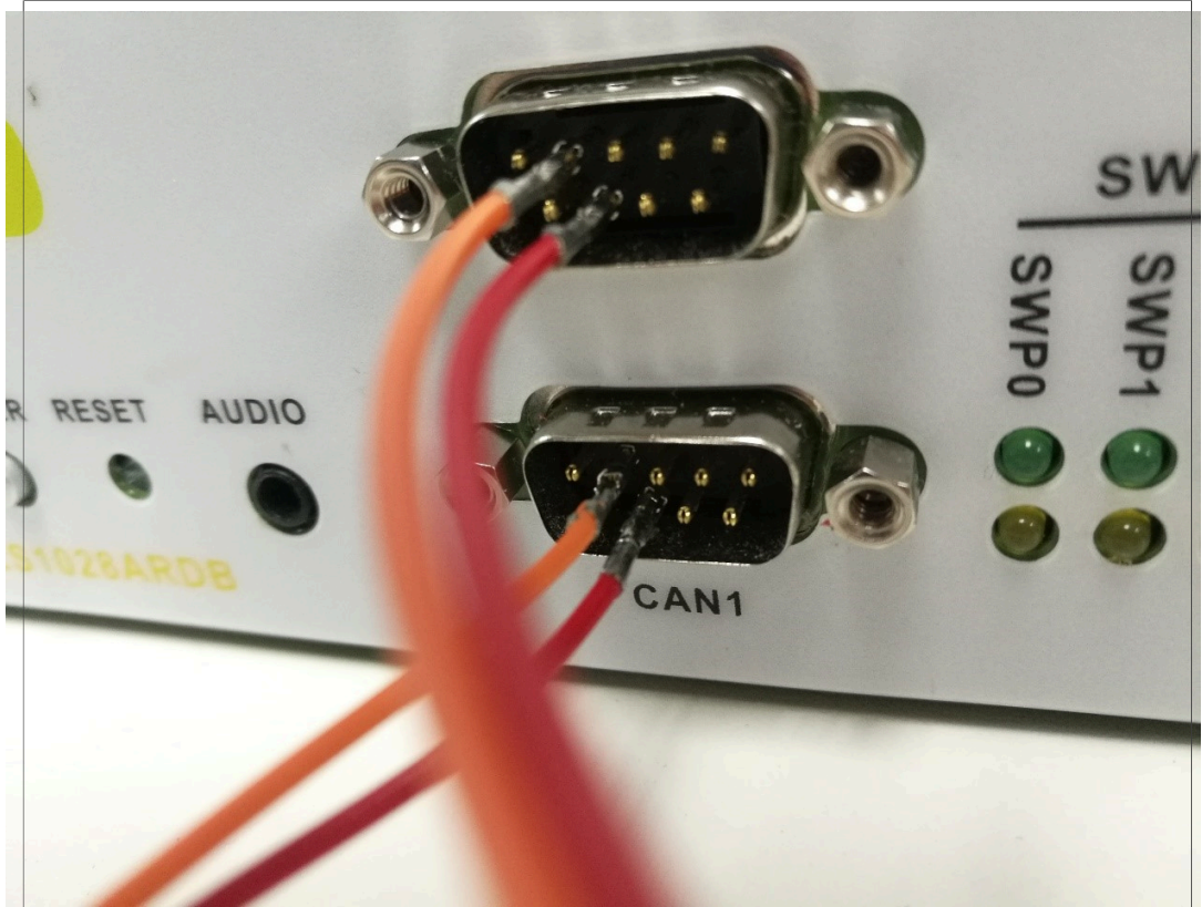
Figure 88. Physical connection for CAN using LS1028ARDB
